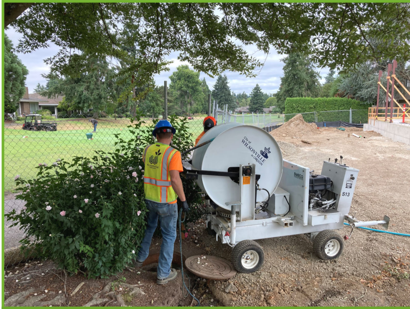
Cleaning sewer mains at the Charbonneau Golf course
