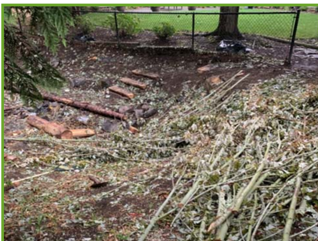
Debris in detention pond
