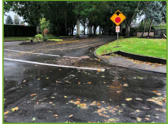
After clearing curb inlet
