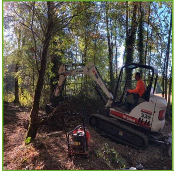
Using an excavator to move dirt
