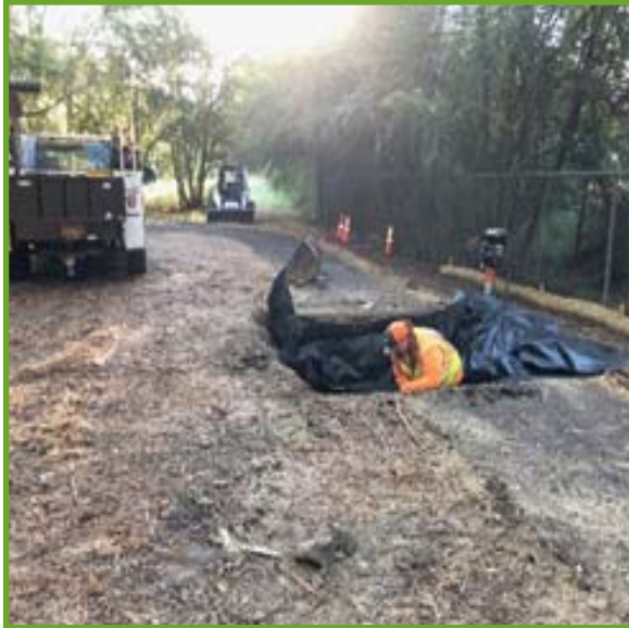
Digging by hand
