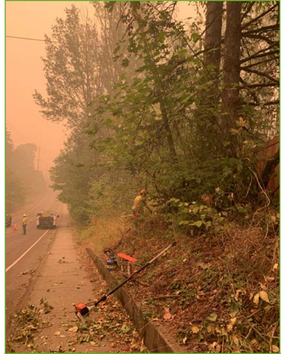
Clearing potential hazards
