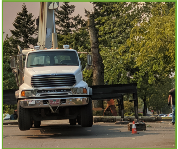
Tree removal at Public Works
