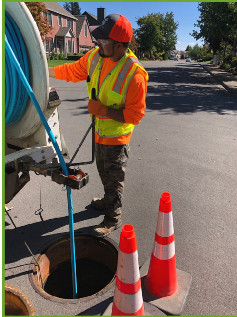
David cleaning a sewer main
