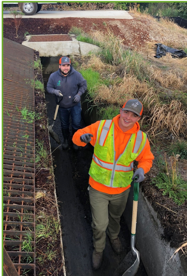
Roman and Konnen cleaning out level spreader
