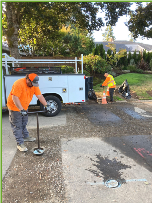
Chad & David shutting off a water main
