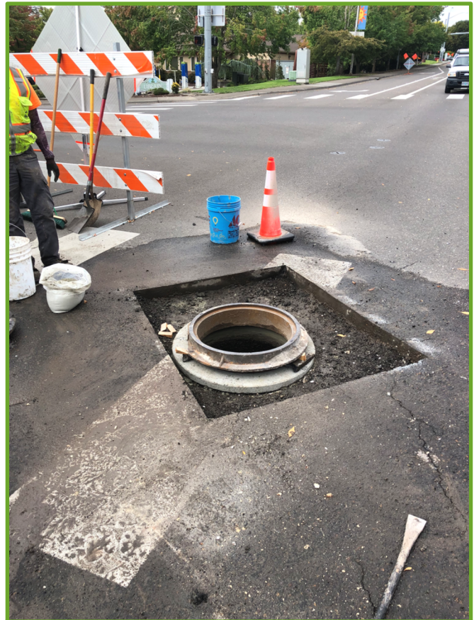
Excavated stormwater manhole
