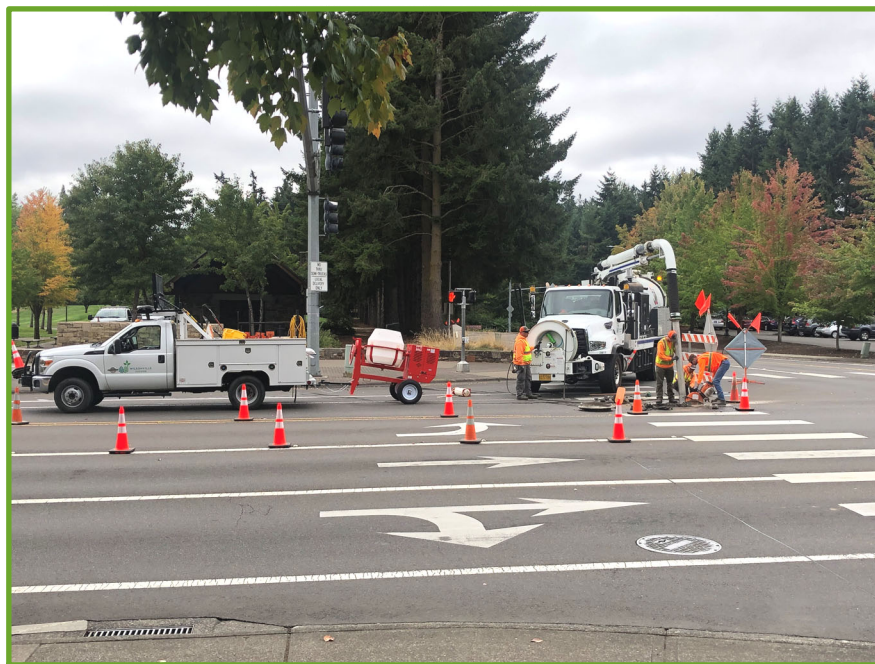
Traffic control for the work site
