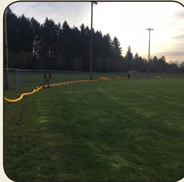
Installed safety cap for Field 4 outfield fence
