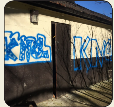
Cleaned up graffiti at River Shelter restroom
