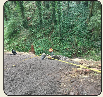
Investigated and began preparations to prepare storm outfall and WTP Park
