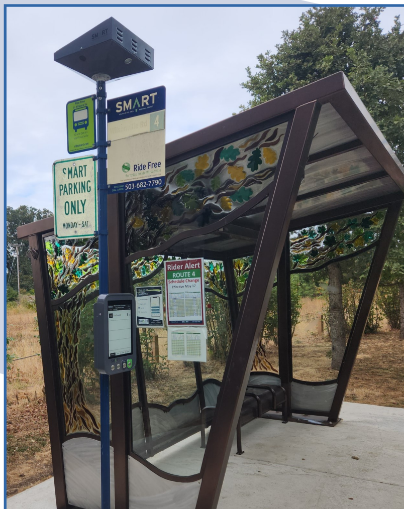
Completed installation, including solar recharge option (solar on top of sign pole)
