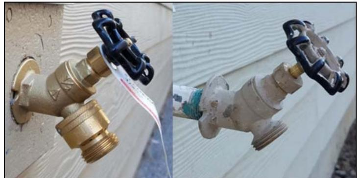
The most common way to prevent the danger of contamination is to install a Backflow Prevention Device that is properly fitted to match the danger. Even a simple hose-bibb can be protected with a vacuum breaker which prevents water back-siphoning as shown in the first photo above. Another very common example is the Double Check Valve that separates the lawn irrigation system from the potable water supply that goes to the building.
