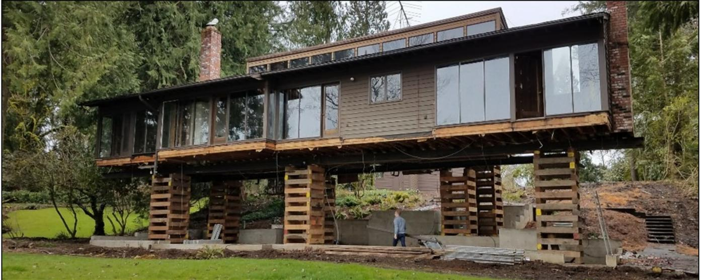
In some cases when construction work occurs in a floodplain, depending on the scope of the project, construction may need to be elevated to a point that is a minimum of two feet above the finish floor, or alternatively the construction must be “flood-proofed.” Generally flood-proofing is much more expensive and difficult to achieve and most folks choose to elevate.
