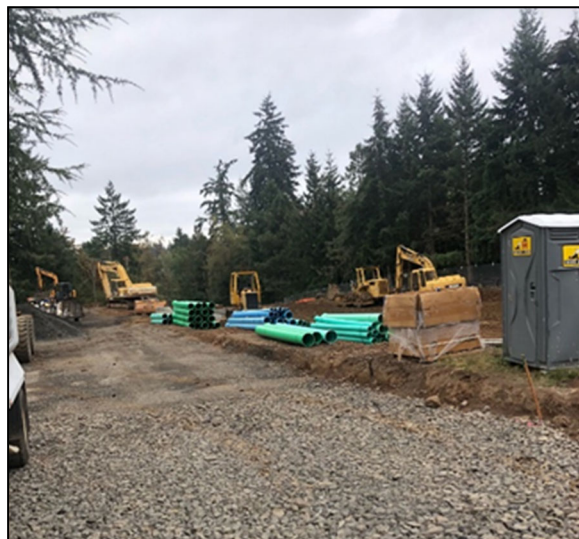
Canyon Creek South Phase 3
