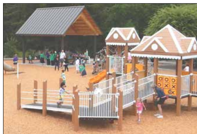
The new accessible play structures installed at Murase Plaza.
