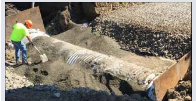
Construction worker spreads gravel over a culvert that runs underneath the Kinsman road extension project.
