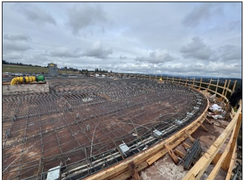
Reservoir roof construction
