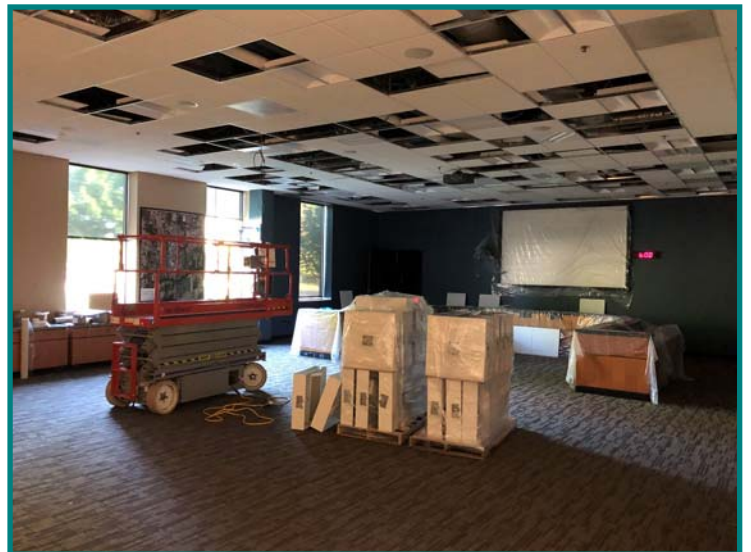
During Project Construction - Council Chambers
