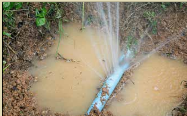
Spring has sprung. Has a leak? The City recommends that residents inspect irrigation systems before regular use. Early detection can lower water usage charges.
