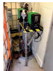
Polymer injector/mixer #3
