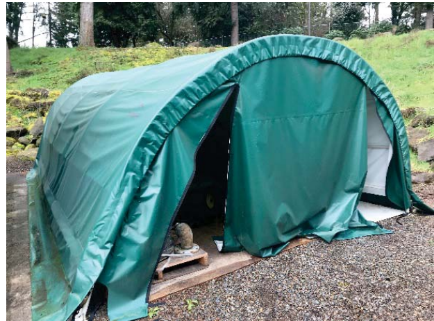
Temporary storage facilities
