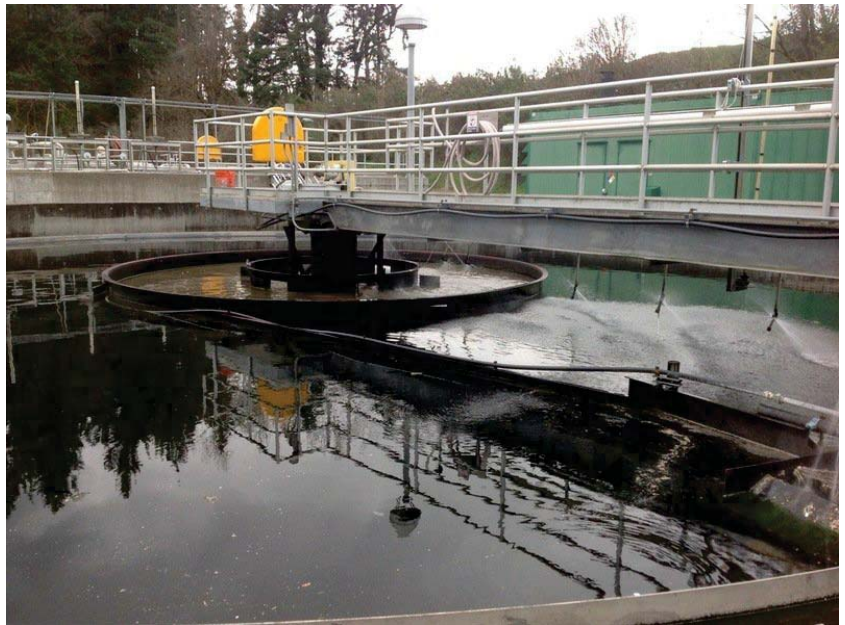
Weir Washer not working
