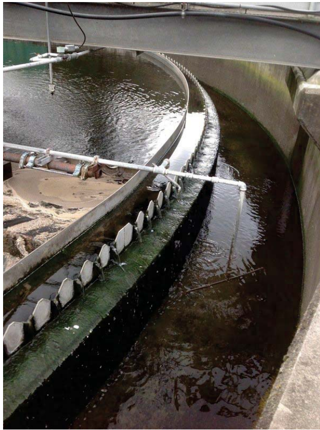
Weir Washer not working
