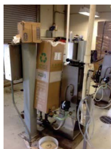
Polymer injector/mixer #1
