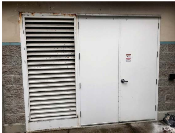
Operations Building door and louver
