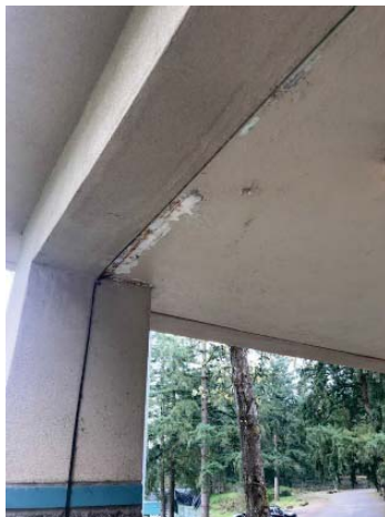
Operations Building ceiling
