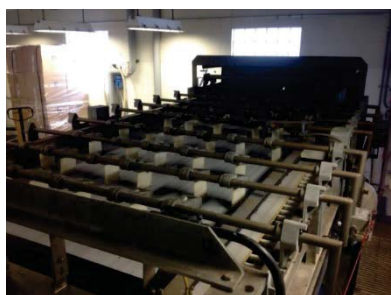
Gravity belt thickener 1
