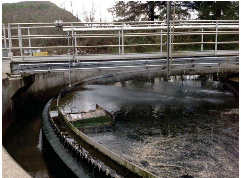
Weir washer not working
