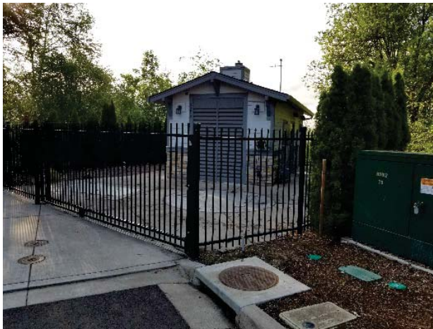
Lift station structure
