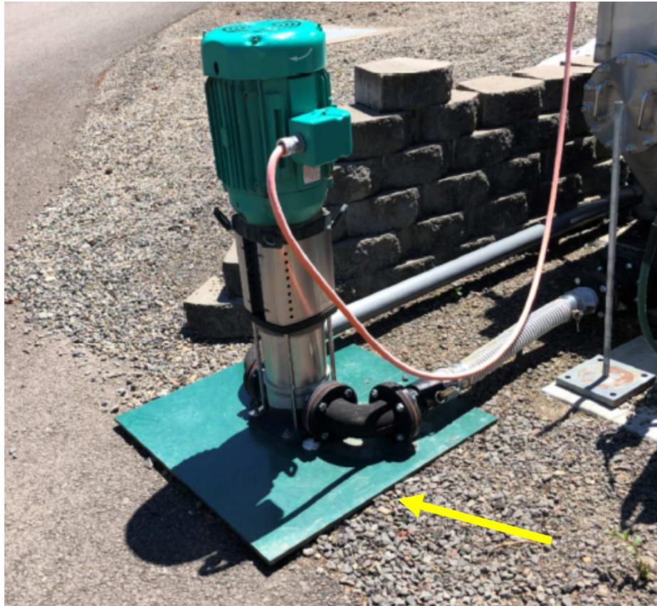
Figure 30 Disk Filters - Recirculation Pump Lacking Resistance to Overturning
