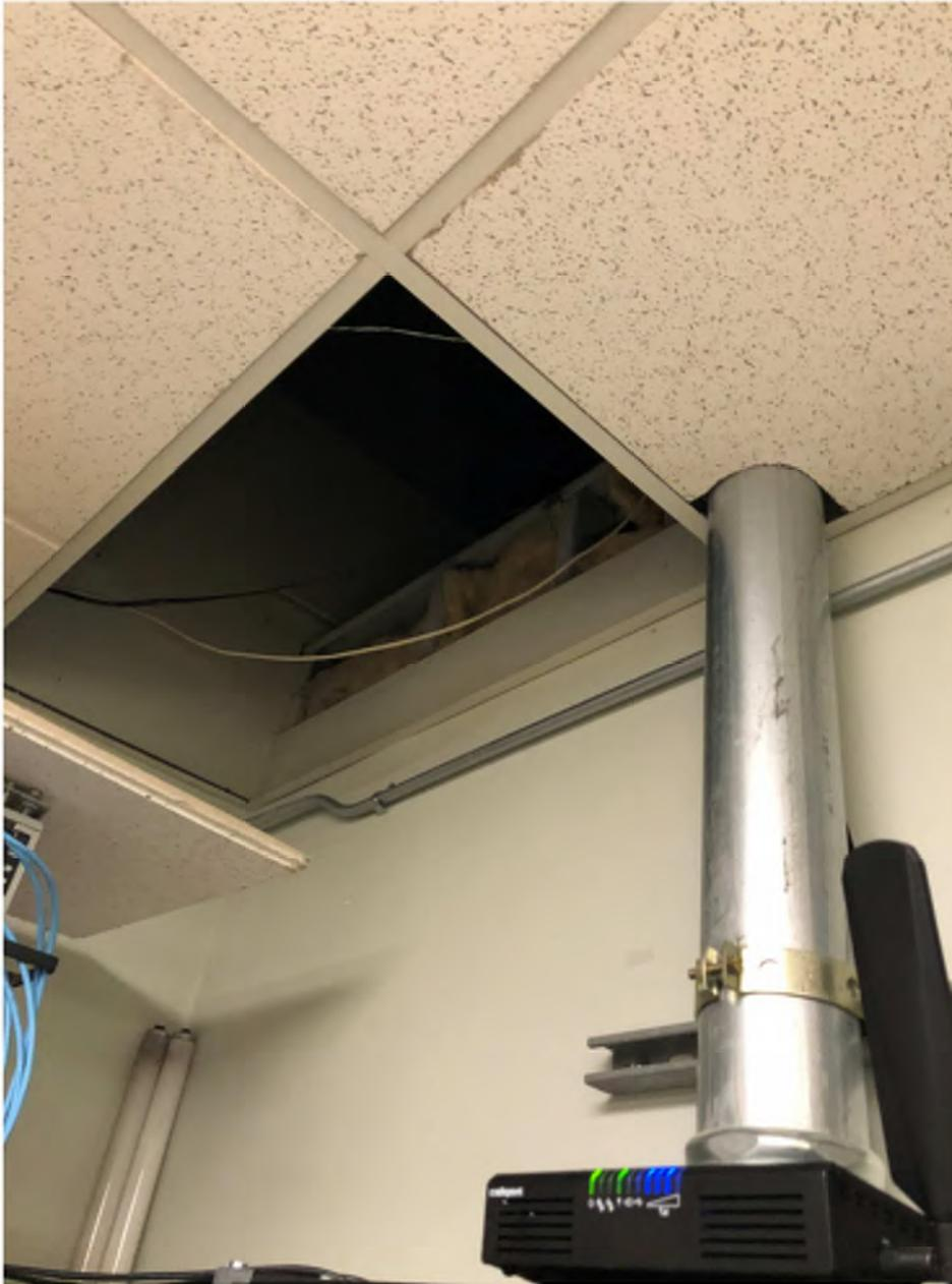
Ceiling supported off wall. There is no gap between ceiling channel edge and wall.
