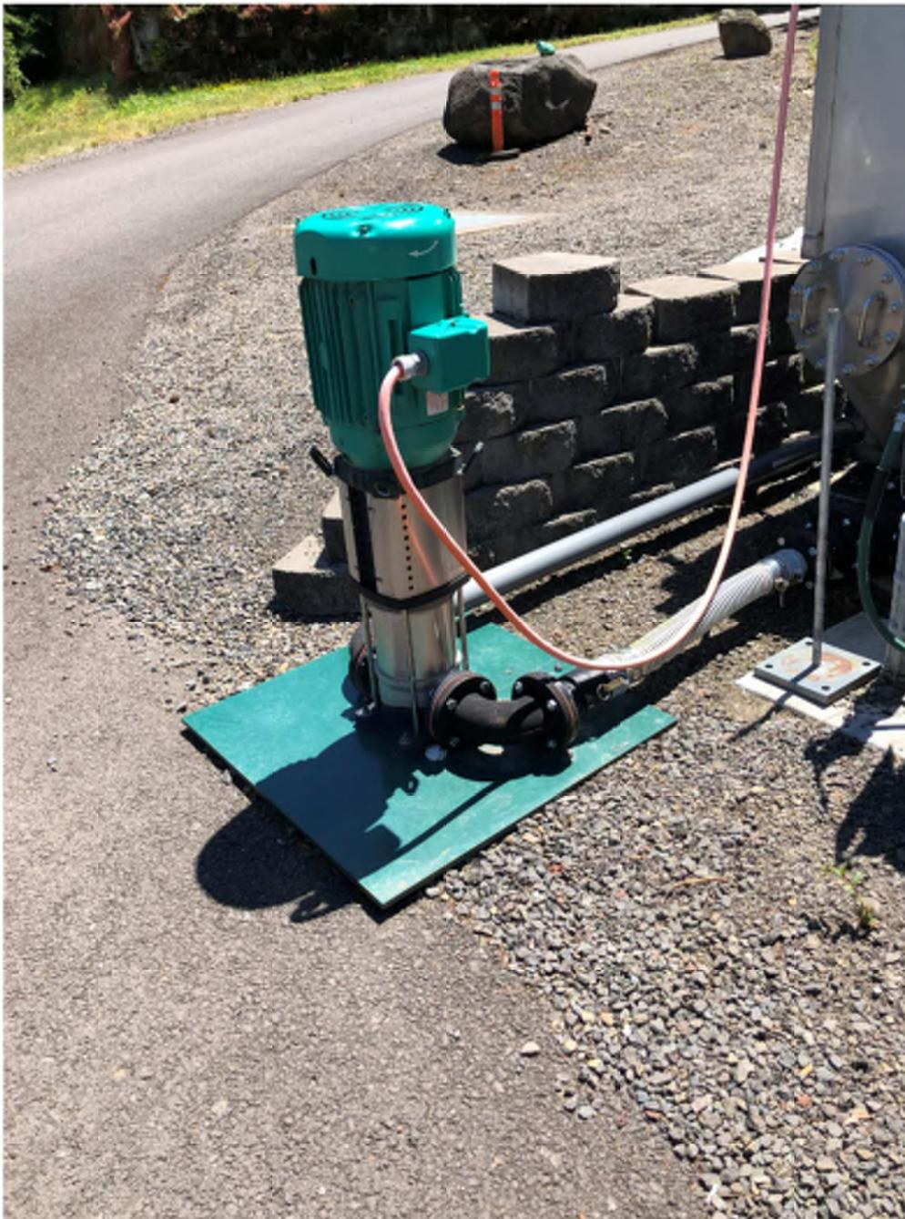
Recirculation pump is anchored to plate below, but there doesn't appear to be any support for equipment overturning.
