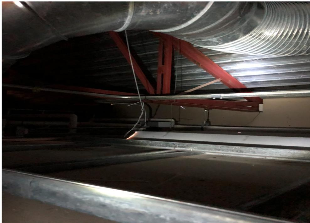
Figure 2 Operations Building - Roof Joist Framing
