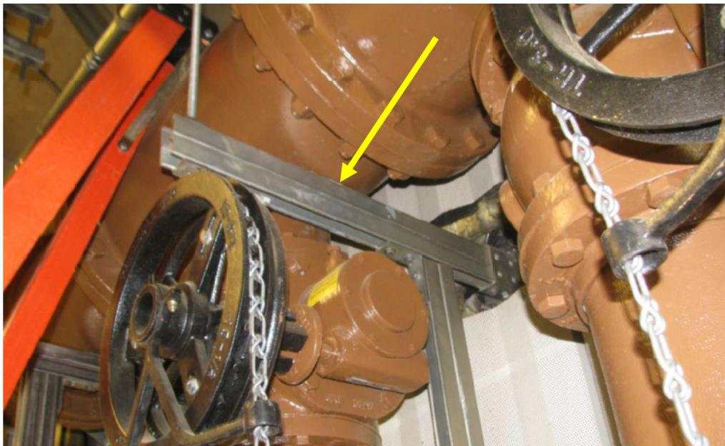
Figure 16 Process Gallery - Piping Lacks Connection Back to Supports Below
