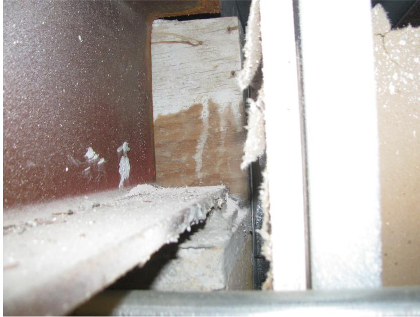
Figure 9 Operations Building - Collector Beam Connection to CMU Wall
