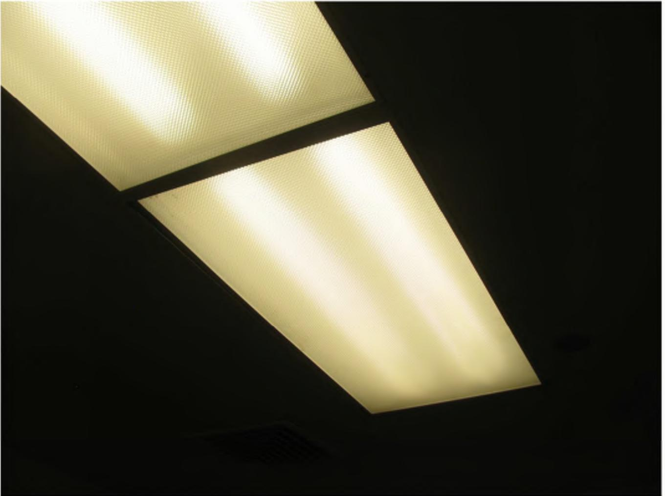
Lens covers within building lack safety devices. The covers currently can swing open without a latch.
