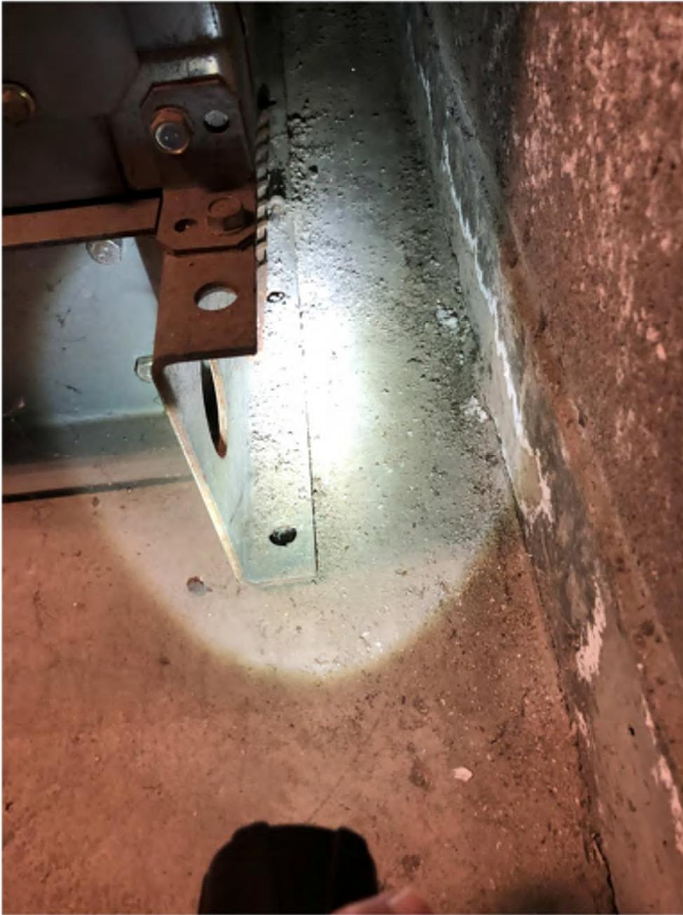
HVAC equipment is unanchored to structure along backside.
