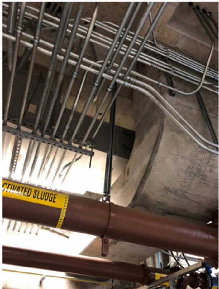
Compression strut lacks diagonal bracing.
