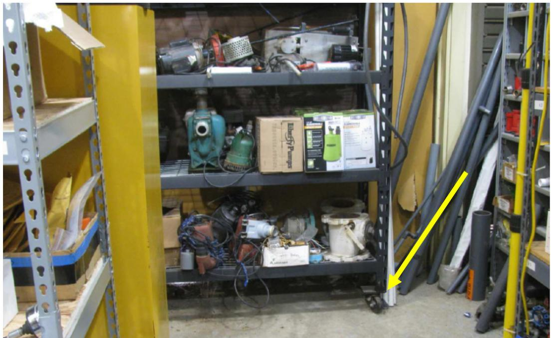
Figure 22 Workshop - Storage Shelving Lacks Restraint to Structure
