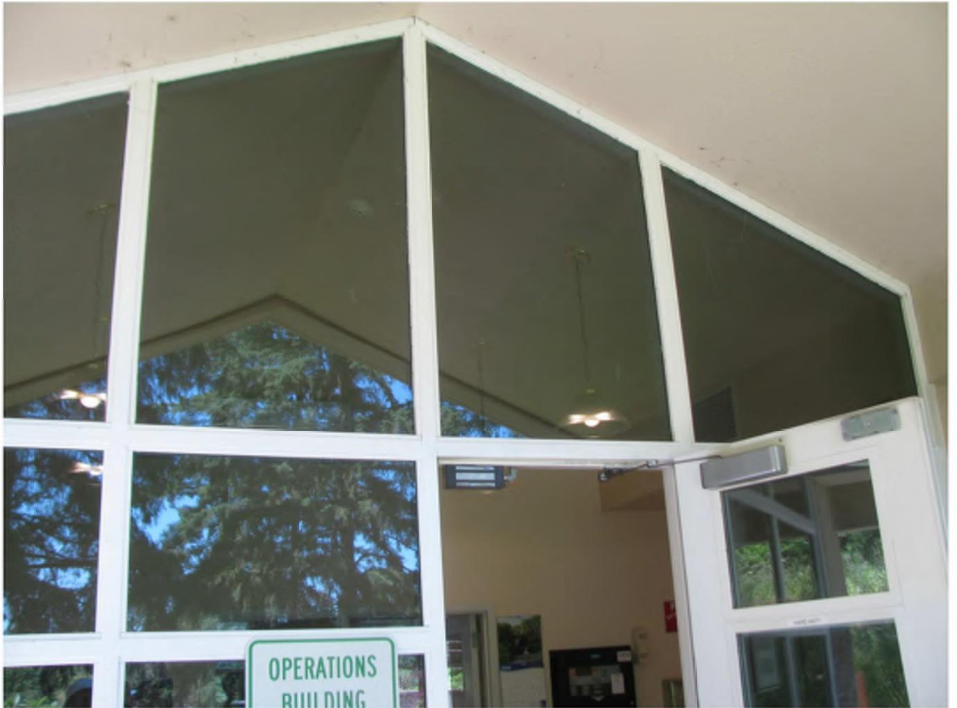
Exterior windows do not appear to meet requirements of heat laminated or have restraint to remain within frame if cracked.
