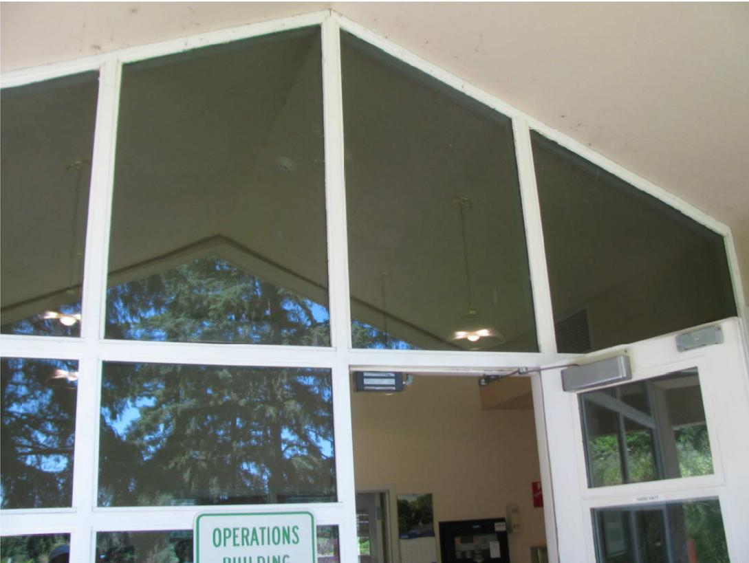
Figure 8 Operations Building - Window Above Entrance Appears to Lack Special Treatment to Limit Damage
