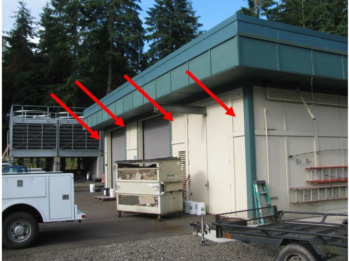
Figure 21 Workshop - East Elevation Shear Walls are Considered Narrow and Could Limit Strength
