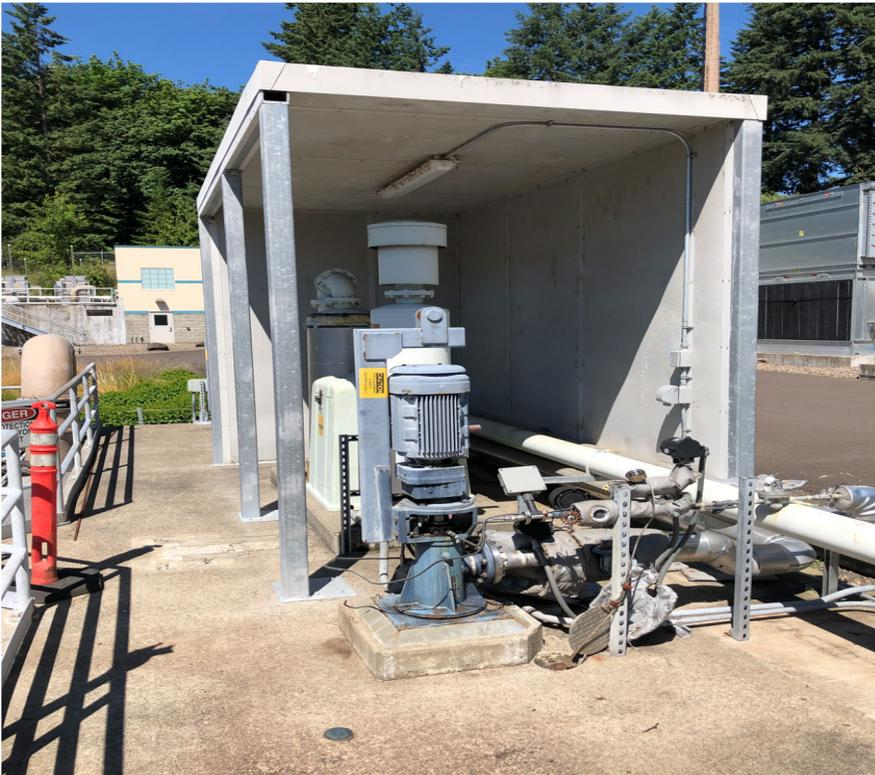
Figure 28 Sludge Storage and Biofilter Basins - Pump Equipment
