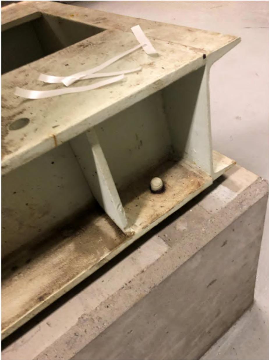
Aeration blower pump lacks anchorage to structure. Nuts are missing or backing off from threaded rods.
