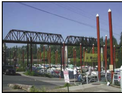
Railroad bridge from Marina
