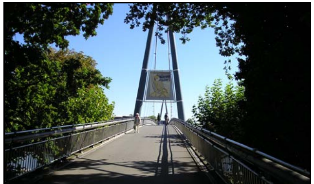
Bicycle/pedestrian suspension bridge in Frankfurt, Germany
