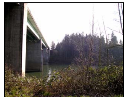
West side of I-5 bridge
