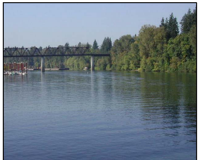
Railroad bridge spanning the Willamette River
