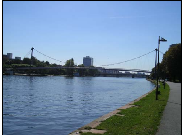
Bicycle/pedestrian suspension bridge in Frankfurt, Germany
