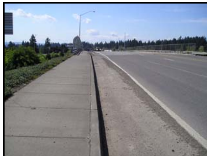
Elligsen Road overpass
