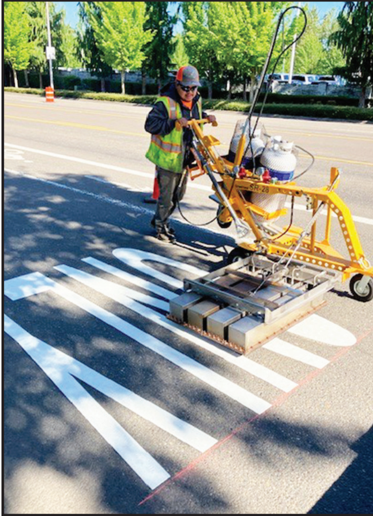
Roads staff refreshing thermal plastic pavement markings.
