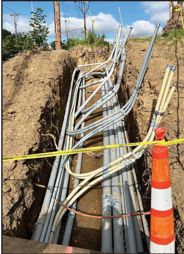
City fiber conduit in the utility trench along Boeckman road (CIP #8093).
