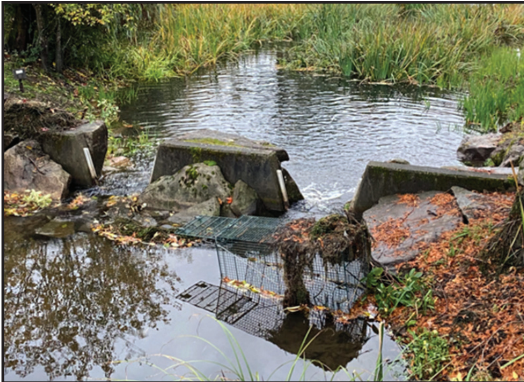
Existing weir system on the Siemens property that will be modified to improve drainage to the Ash Meadows area. (CIP #7068).
