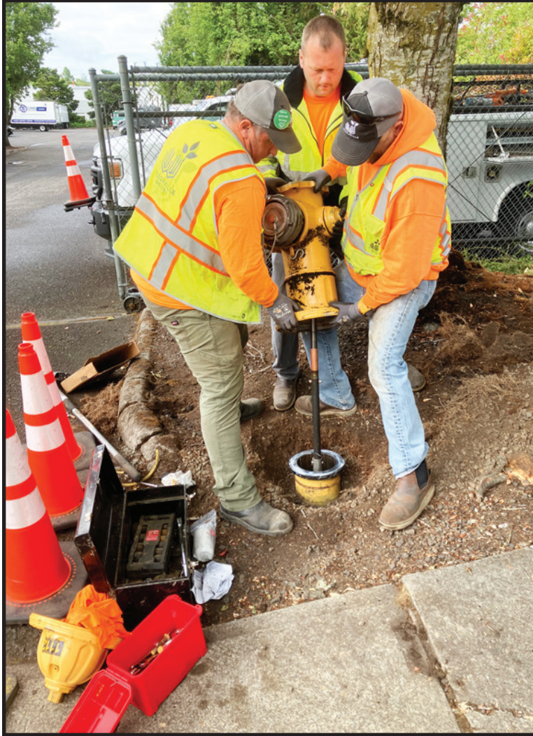
Utilities Technicians use teamwork for heavy lifting jobs to replace fire hydrants.
