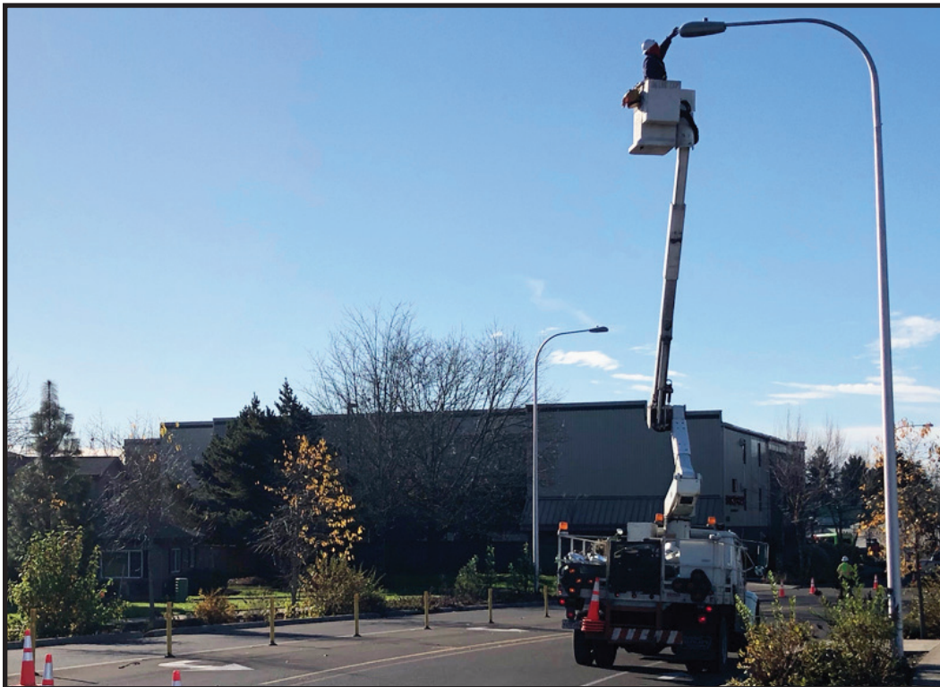
LED streetlight conversion project - light installation.
