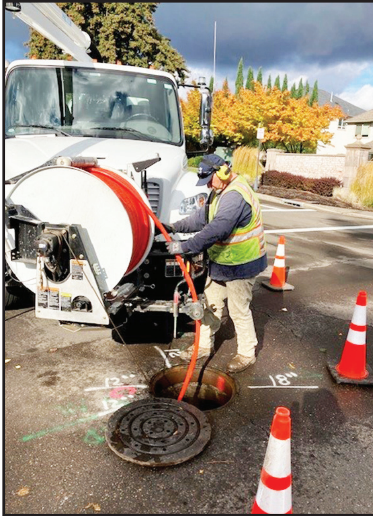
Stormwater staff performing storm system cleaning and CCTV inspection.
