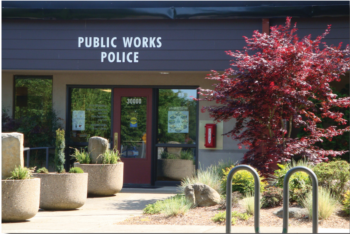
Public Works/Police Building
