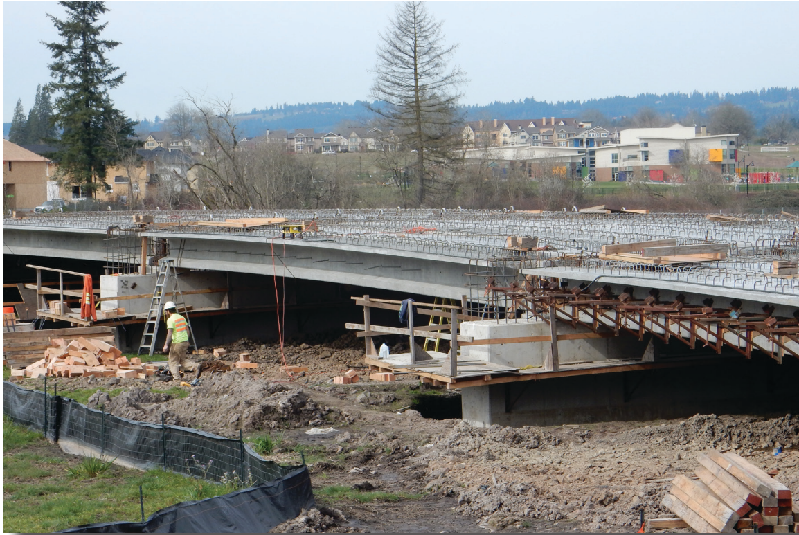
Barber Street Bridge Extension
