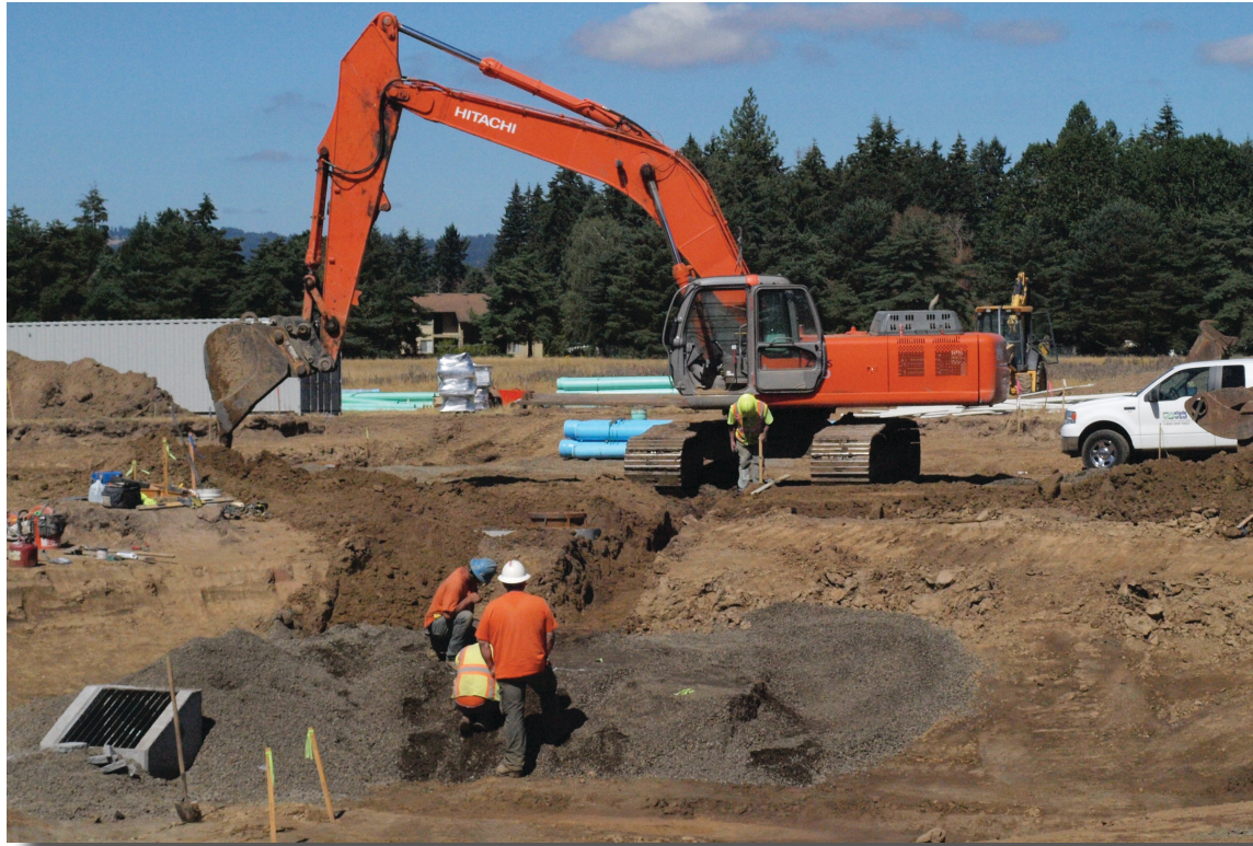
Villebois Construction Site
