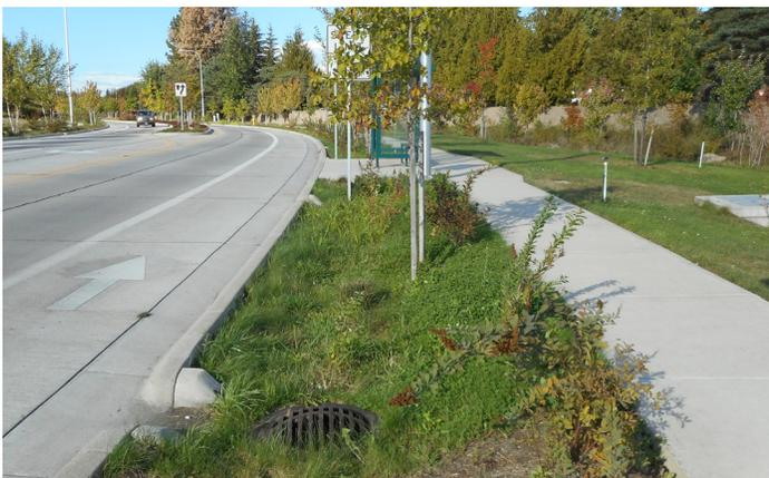
Example of vegetated swale to manage roadway runoff.
