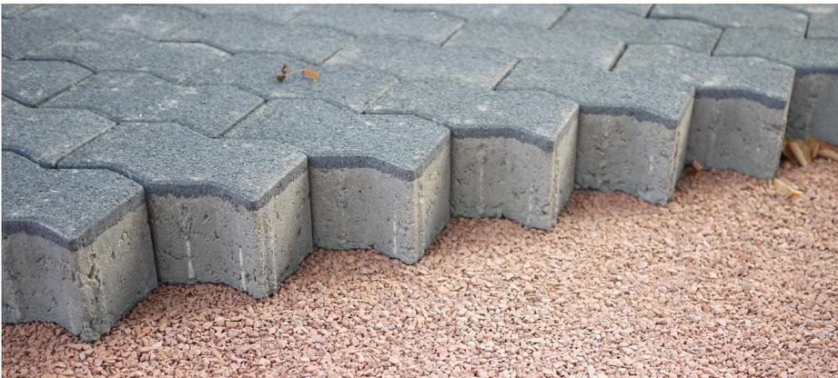
Gaps in the pavers allow water to soak into the ground.
