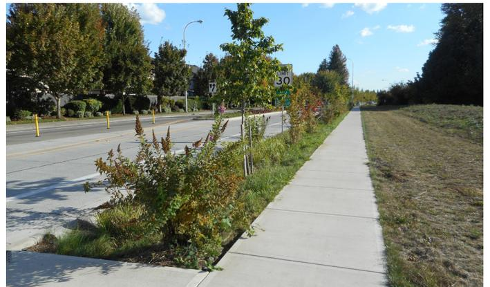
Roadway embankments and sidewalks provide opportunity to install filter strips to treat runoff from adjoining impervious areas.
