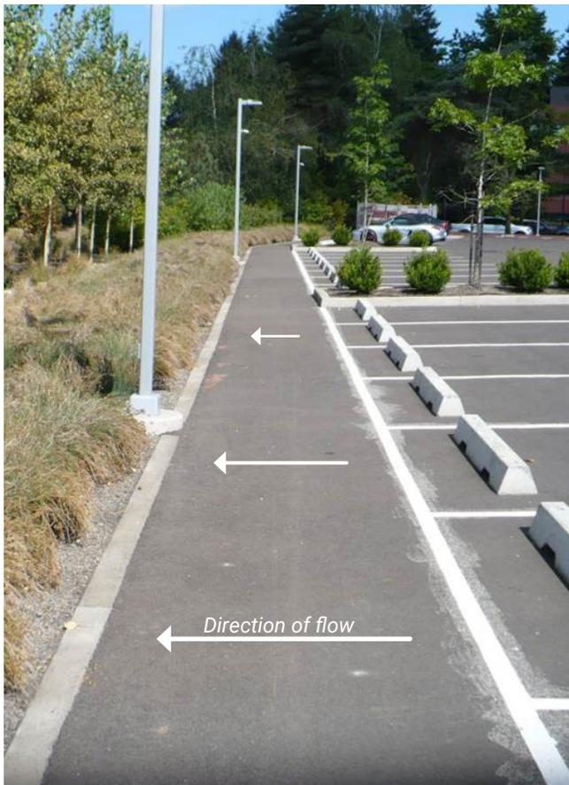
Integrating filter strips with parking areas helps to manage stormwater at the source.
