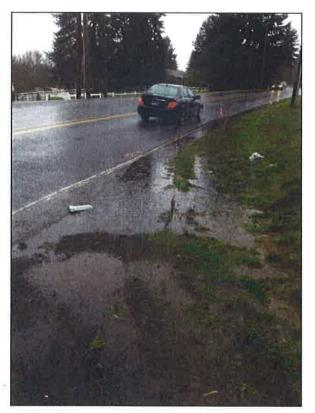
**Photo C2.** At top of photo is the original Washington County culvert outlet under Boones Ferry Road discharging to the west (December 2012). This is an old concrete pipe. The pipe at the lower-left portion of the photo is the plastic pipe draining onto the Lucini property.
