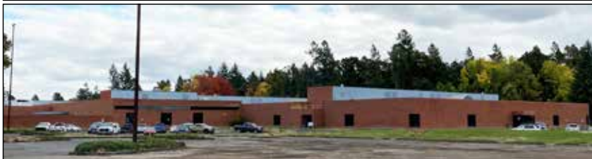
California's Twist Bioscience is investing $70 million to transform the 190,000-square-foot ParkWorks Industry Center (bottom) into a state-of-the-art factory that manufactures synthetic DNA. The move is expected to bring 400 new family-wage jobs to Wilsonville.
