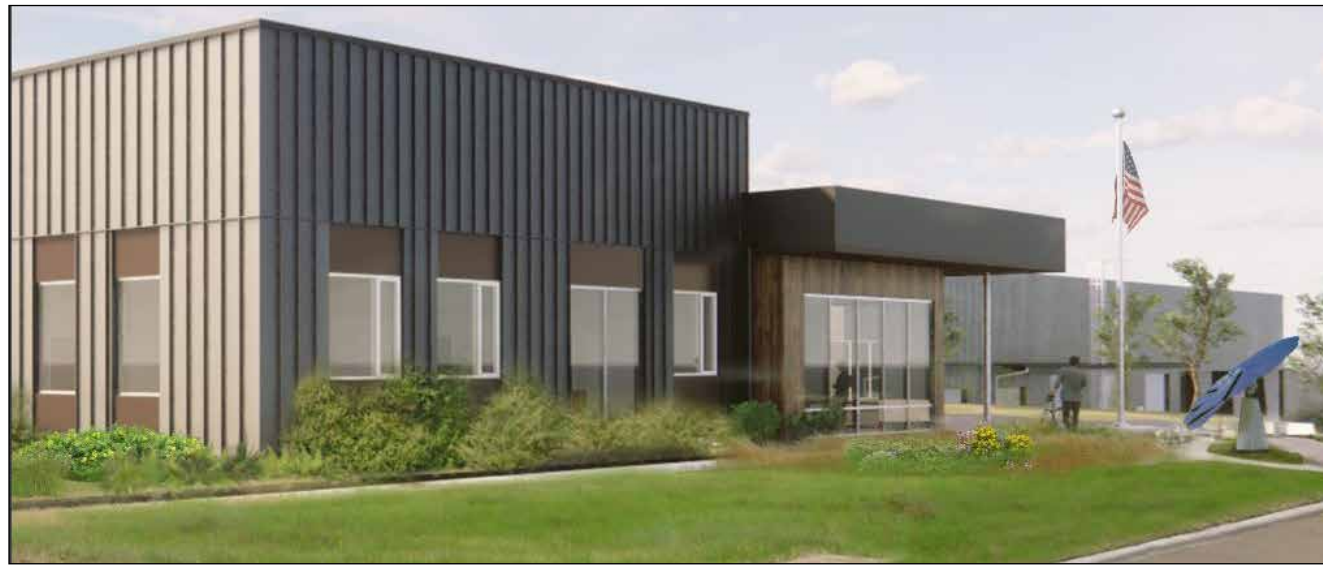
Centrally located north of the SMART Transit/Fleet offices on Boberg Rd., the City's future Public Works Complex centralizes operations and is to serve as the City's Emergency Coordination Center.
