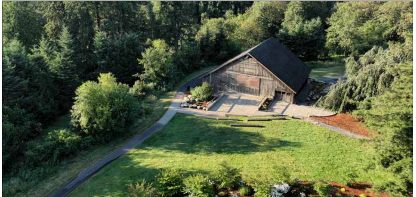
Parks maintenance staff has worked to provide a more private and intimate setting for the many weddings and social events held at the Stein-Boozier Barn at Memorial Park. The City is hosting a spring open house to showcase the facilities.
