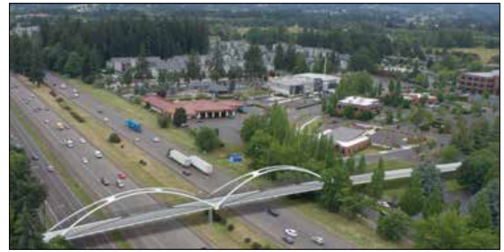
This rendering demonstrates how a “tied arch” bridge might look spanning over Interstate 5 near Wilsonville Town Center.
